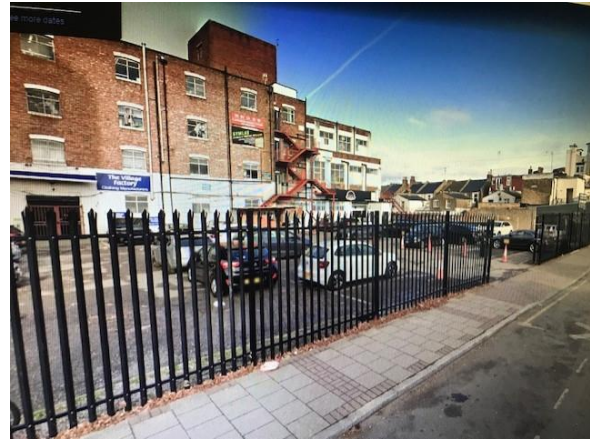
Cypress House Car park at the rear
